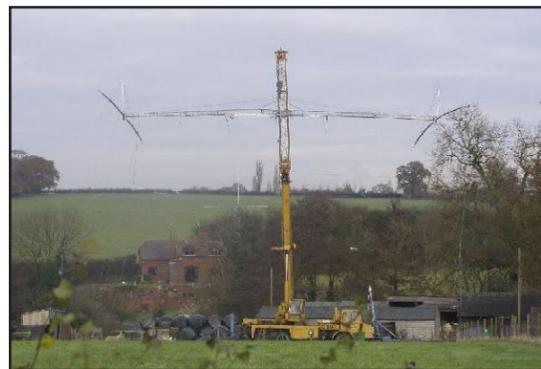
Yagi-Uda for 160/80/40m belonging to Dave, G0EVY with crane rotor. The massive array is homebrew and tips the scales at over 1000 pounds! Photo by Dave, G0EVY.
